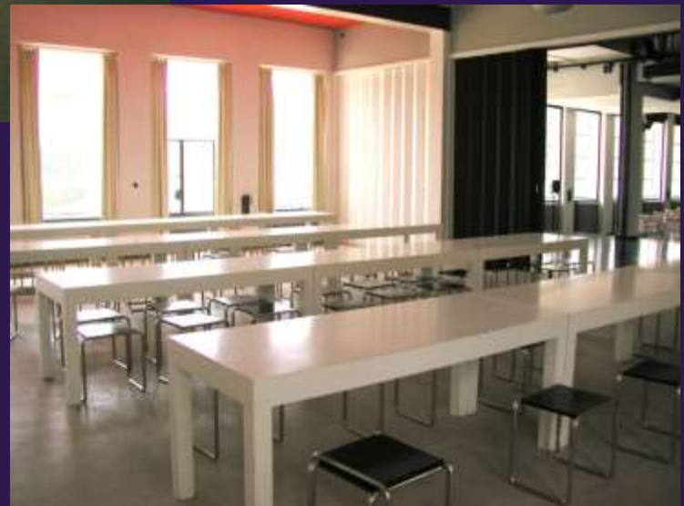
Ceiling with light fixtures for stage
