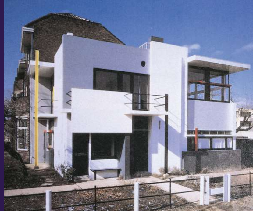
Gerrit Rietveld, Schroder House , 1924, Utrecht, Netherlands
