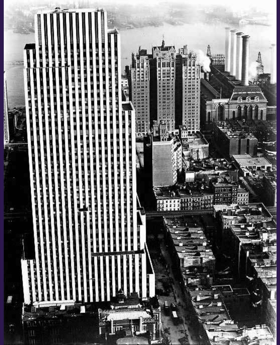
Raymond Hood and John Mead Howells, Daily News Building ; 42nd Street between Second and Third Avenues, New York, 1929-31
