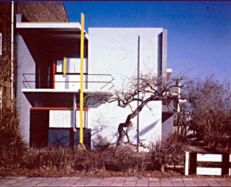
Gerrit Rietveld, Schroder House , 1924, Utrecht, Netherlands
